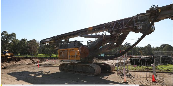
The piling rig on the construction site drilled 45 holes, with a total of over 360 metres dug across the site.
