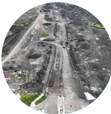
Drone images of progress on Edgars Road
