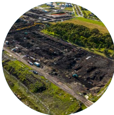
Habitas civil works
