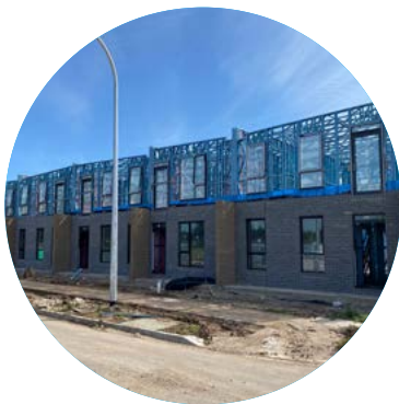
LUMA Stage 1 construction underway
