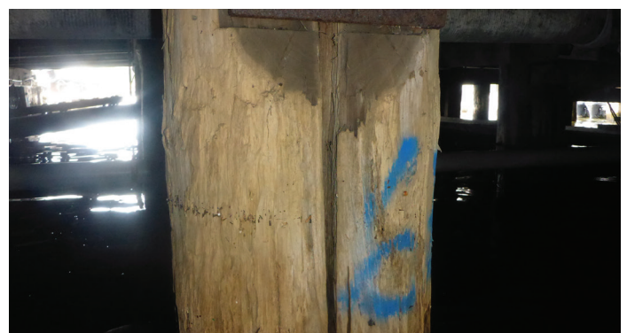
Split pile Wharf 9
