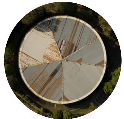
The decommissioned water tank
