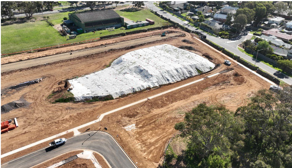
Existing covered topsoil stockpile, Riverwalk, Werribee
