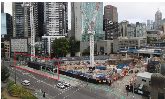
Gantry install along Southbank Boulevard
