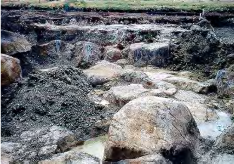
Figure 1: Example of excavation for spread footing supported on basalt
