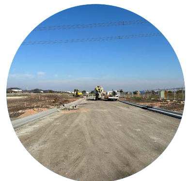
Berrigan Street & Herlitz Drive extension works
