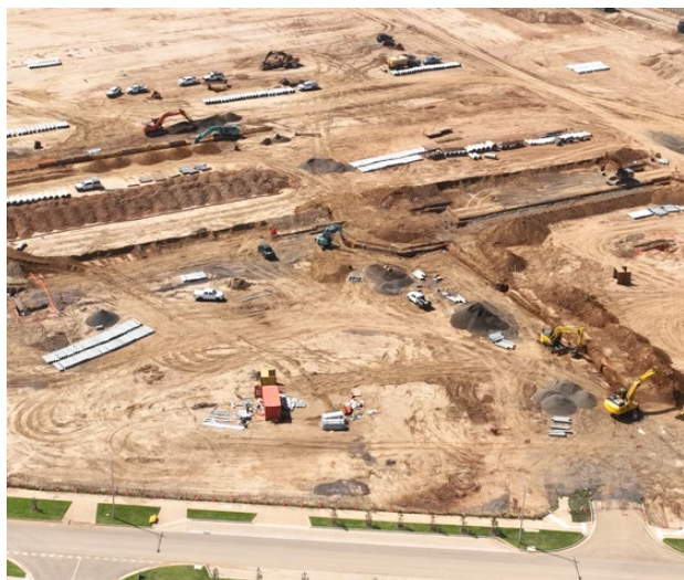
Earthworks and civil works in stages 42 – 47
