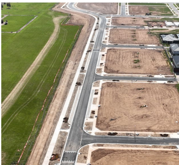
Civil works in stages 37 & 41
