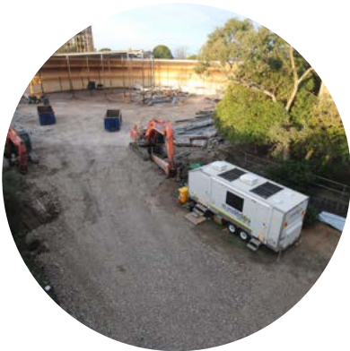
Current works underway to remove the walls
