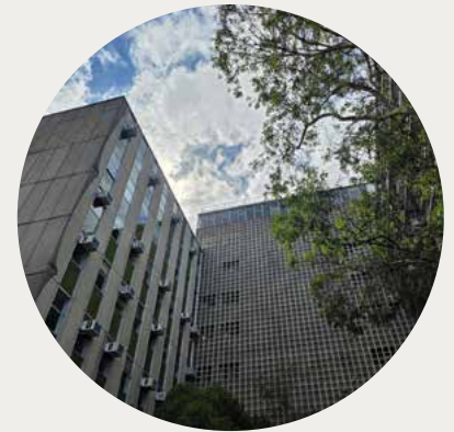
Southern building on Denmark St
