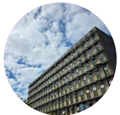
Southern building on Denmark St
