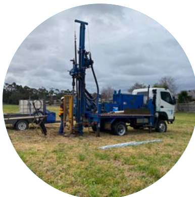
Images show our Geologist inspecting the soil samples taken and the drill rig used to complete the investigative works
